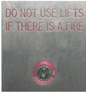
Figure 1 Recall Fire Service switch
